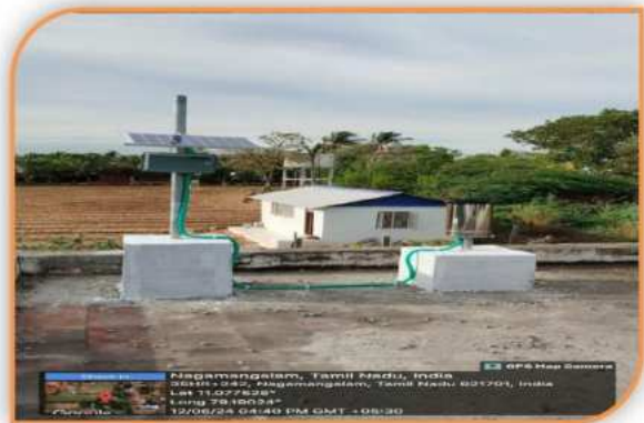
ARG02 – Nagamangalam(E-seva Building)
